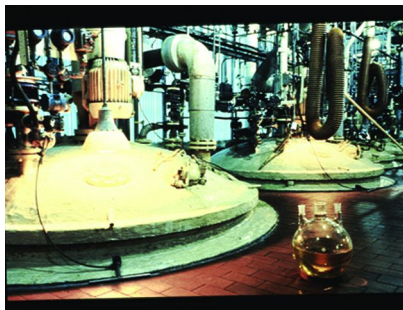
Figure 2. Lab to plant scale-up. (Courtesy of the author.)
